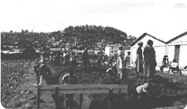
ANOSIBE COMMUNITY HAND DIGGING STAGE ONE FOUNDATIONS MAY 2007
