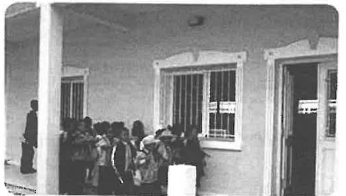
NOVEMBER 2007, PERMANENT CLC-ANOSIBE FACILITY STAGE ONE IN FULL USE.
