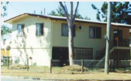
Gable low pitch, vermin proof flooring (studs not mortice and tennon into bearers), panel cladding, on stumps
