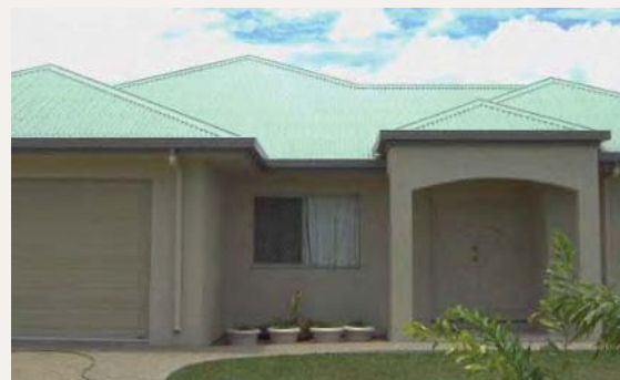
Reinforced masonry block, hip and gable, large truss spans, medium roof pitch, slab on ground
