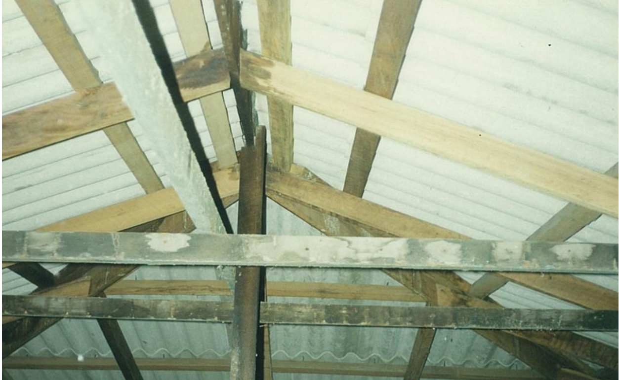
Figure 7. Example of typical pitch frame construction (pre-1960s)
