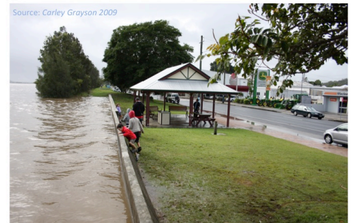
Source: Carley Grayson 2009 Permanent Flood Barriers in Maclean, NSW prevent frequent catastrophic flooding of the town centre
