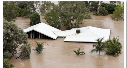
A preventable risk? - Landuse planning regimes do not always prevent inappropriate development or stipulate building methods that are resilient.
