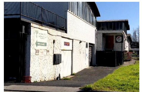
The visibility and appeal from the street is poor and uninviting. The modernisation of the space is well overdue.
