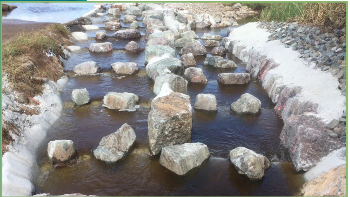
Tedlands Barra ladder during flow
